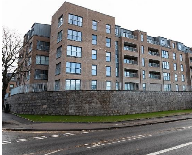
Buff brick used at former Craiginches prison site
