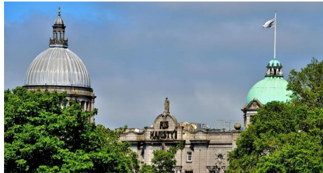
St Mark's Church (left) and His Majesty's Theatre (right) have lead and copper domes respectively
