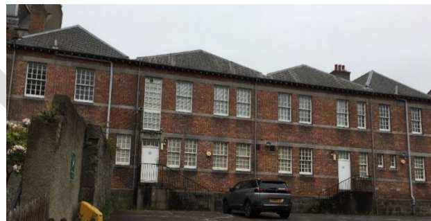
Red brick rear façade of 111 Gallowgate
