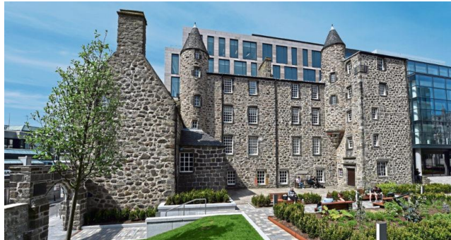
Provost Skene's House – Built of granite-rubble in the 17 th century it is one of Aberdeen's oldest remaining buildings
