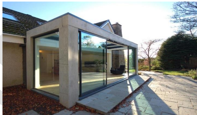
The use of glass in this house extension maximises daylight receipt and minimises the extension's massing
