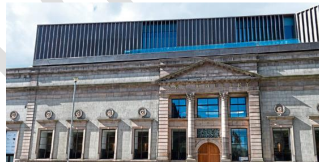
The red/brown colour of the Art Gallery roof extension reflects that of the pink Corrennie granite below.
