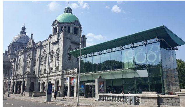
The green-tinted glass extension to His Majesty's Theatre reflects the colour of the building's copper dome above
