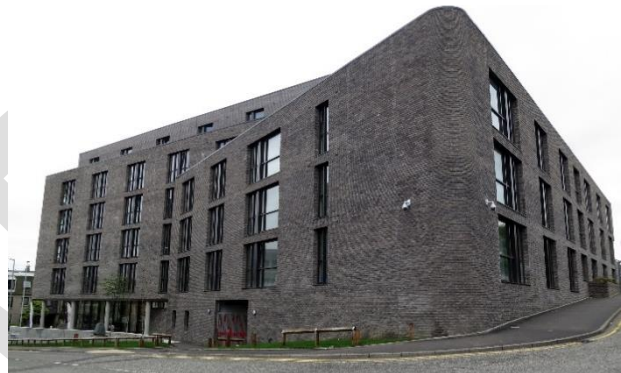
Grey brick used at 2 Powis Place student accommodation
