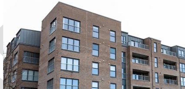
Metal cladding creates a roofscape at Craiginches
