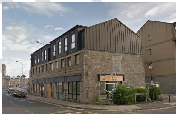
Dark grey metal cladding used to create a roofscape at the former Remnant Kings building on Loch Street
