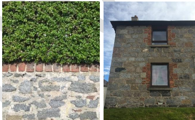
Granite wall with brick coping and window surround detailing – characteristic 'Seaton red'
