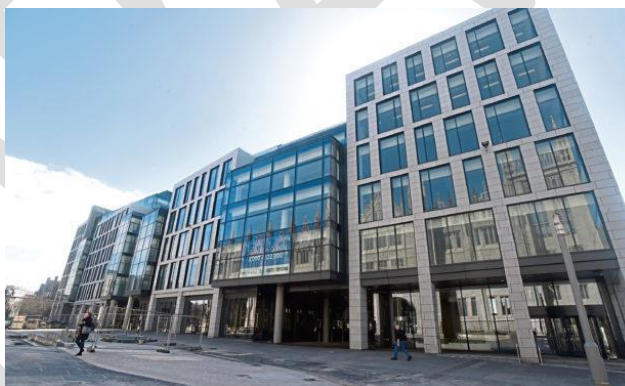
Imported granite cladding panels have been used on new buildings in Aberdeen such as Marischal Square.
